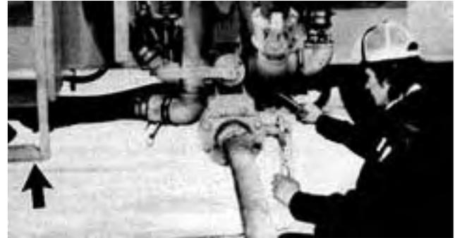
FIGURE 23. Operator Directly Behind Engine Exhaust Outlet when Filling Tank.
